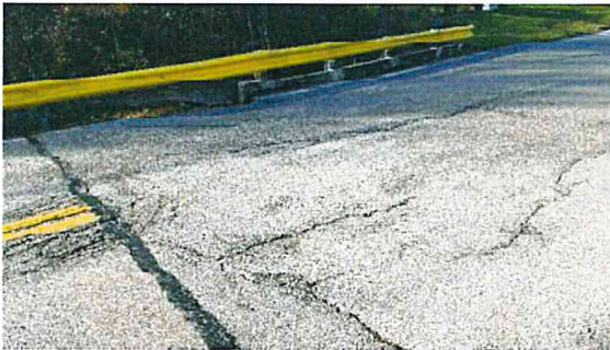
Exhibit 3: Pavement sag at abutment
