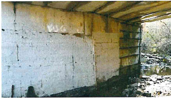
Exhibit 6: East side abutment (Note metal banding, bolts, and grout/paint)
