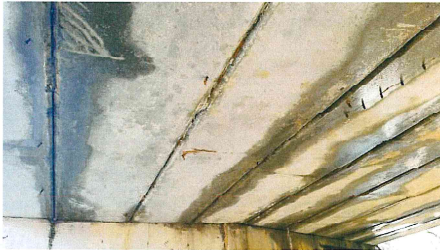
Exhibit 8: Bridge deck and seepage (Crack and epoxy injection tubes present at upper right corner of photo)
