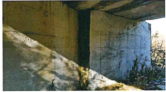
Exhibit 7: West side abutment (Note abutment offset and honeycombing)
